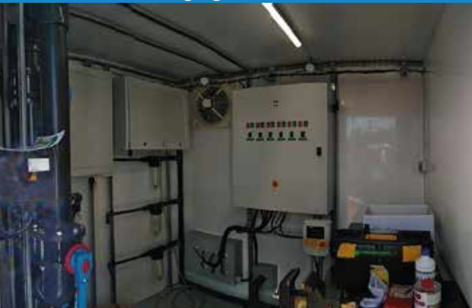
Container with two dosing cabinets - FeCL3 and flocculating agent
