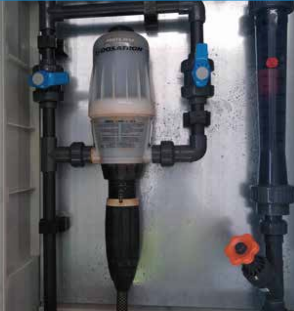
Container with two dosing cabinets - FeCL3 and flocculating agent
