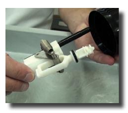
Step 12: Slide the actuator assembly out.
