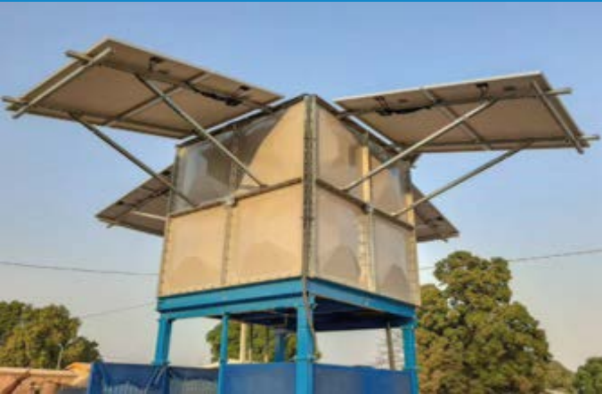
A solar pump station with a capacity of up to 2,480 W
